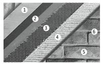
In sequence: (1) sheathing, (2) two layers of water resistive barrier (WRB), (3) galvanized metal lath, (4) mortar, (5) Modulo Brick thin veneer, (6) mortar joint.
