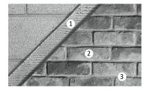
In sequence: (1) mortar applied directly to untreated, unpainted masonry, concrete or stucco, (2) Modulo Brick thin veneer, (3) mortar joint.
